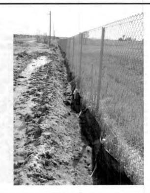
Photo Number Inspection Date Photographer Description 11 6/6/2013 Seth Draper Upgradient and interior view of the construction site. Majority of the stormwater runoff from the construction site travels directly east, toward photographer. SWPP Plan/Site Map shows a temporary sediment basin should be installed. Photo is facing west.
