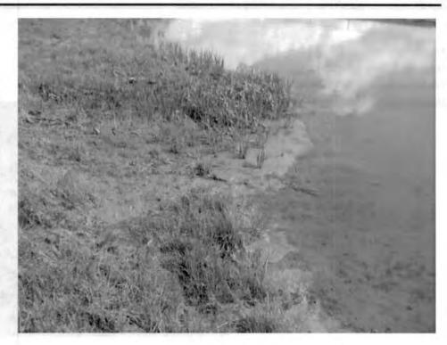
Photo Number Inspection Date Photographer Description 17 6/6/2013 Seth Draper Improperly maintained silt fence located on the eastern border of construction site is shown in photo center. Silt fence shown in photo is the upgradient view of the single line of silt fence shown in photo 14. Photo is facing west.
