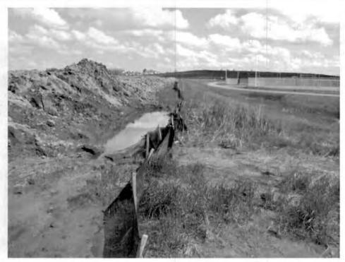
Photo Number Inspection Date Photographer Description 15 6/6/2013 Seth Draper Stormwater that flows over the silt fence in photo 14 flows into detention basin shown in photo center. Detention basin is not part of the construction site. The detention basin shown in photo is part of the Bismarck MS4. Photo is facing northeast.
