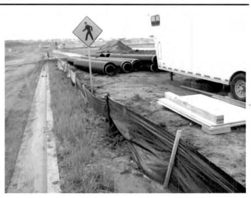
Photo Number Inspection Date Photographer Description 23 6/6/2013 Seth Draper SWPP Plan/Site Map detailed that the site would feature a construction entrance/exit at photo location. No construction entrance/exit was installed at time of the inspection. Note trackout from site. Photo is facing west.
